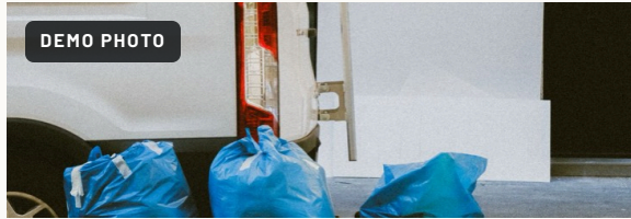
Fig. 9 · Waste removal and HEPA vacuuming
